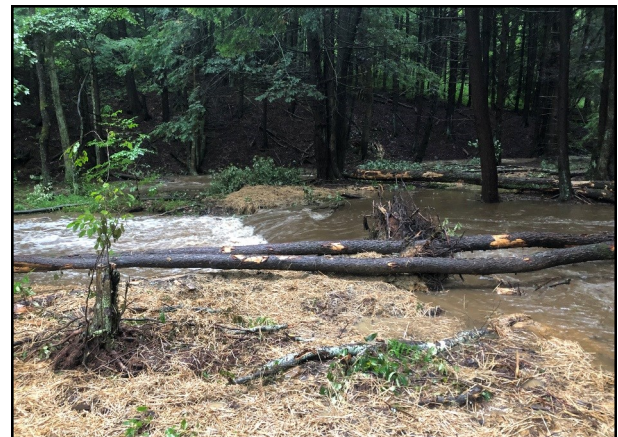
Little Arnot Run during a high flow event post construction. An intense storm dumped nearly 4 inches of water in the region over the course of a day shortly after restoration activities on the LAR floodplain. Removing artificial levees and other earthen barriers to natural flow and installing large logs and wood material to the stream allowed flood-waters to enter and flow across the floodplain.
